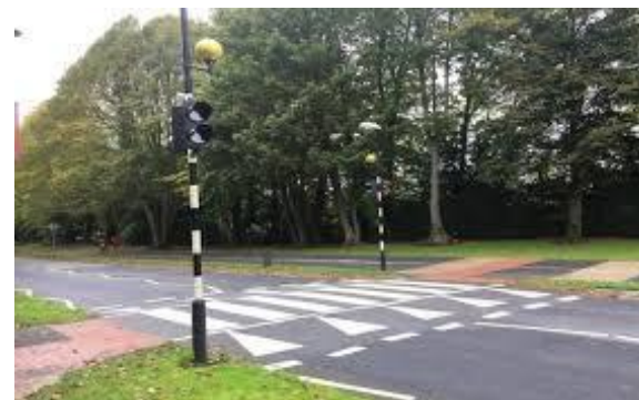
Pedestrian crossing at The Terrace
