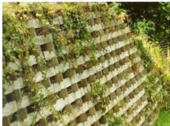
Vegetated timber crib retaining structure
