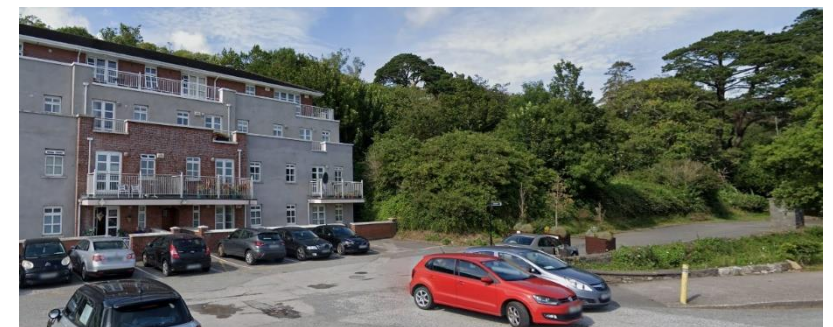
View of lower site from Johnstown Close
