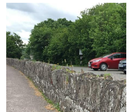
Low roadside wall along car park
